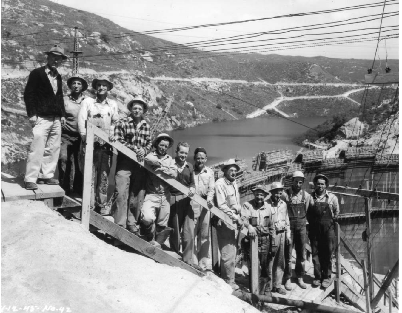
The Loveland Engineers, named for its founder Chester H. Loveland of San Francisco, bought the Sweetwater Water Corporation in 1927 and built the Loveland Dam near Alpine 18 miles upstream from the Sweetwater Reservoir. It was finished July 17, 1945, and at 203 feet high, it doubled the capacity of the Sweetwater system. (Photo from Bonita Museum)
