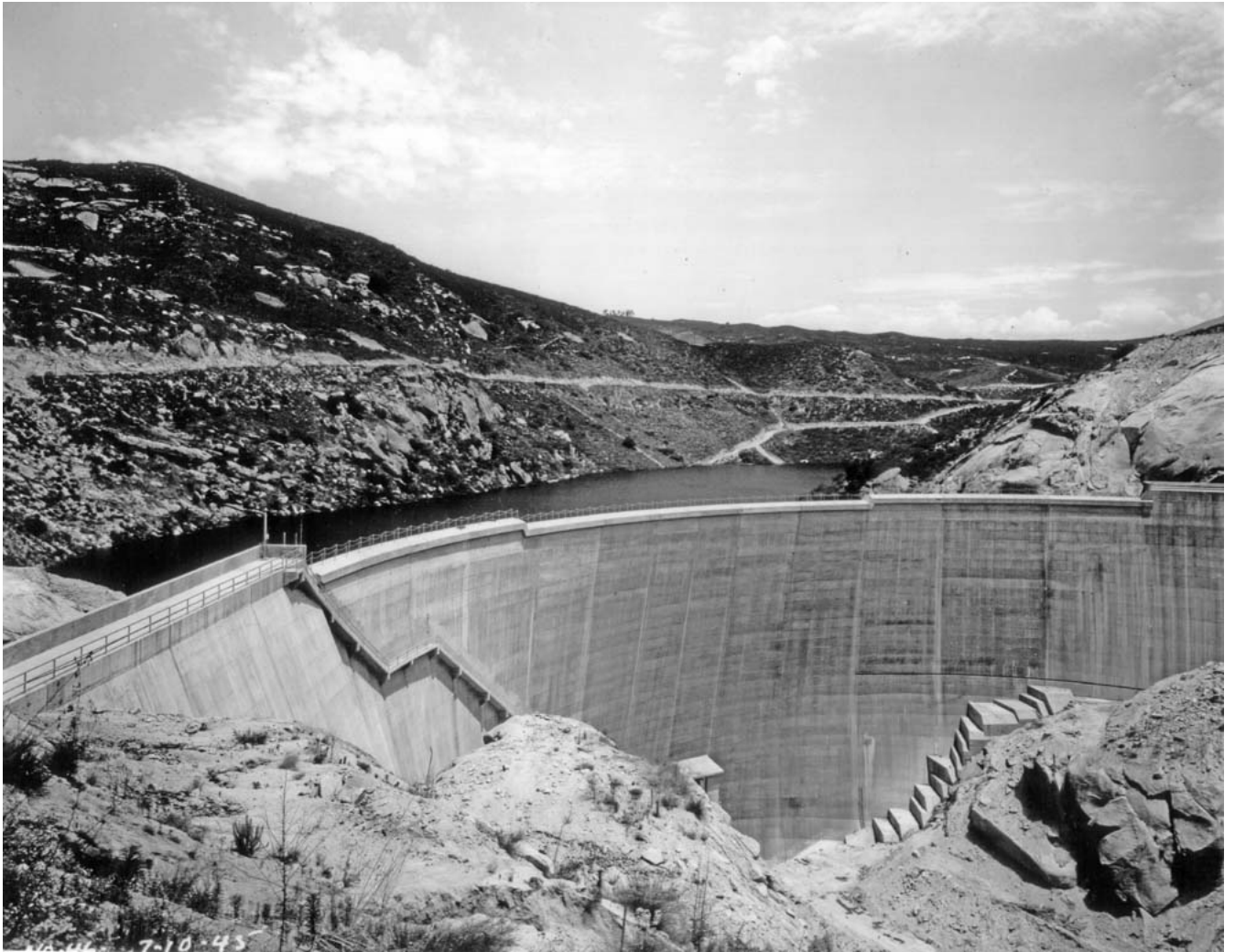
The Loveland Dam, shown here in 1945, was owned by the California Water and Telephone Company, the new name of the Loveland Engineers after 1935. This company was sold to a Delaware group in 1966 and became known as the California Water Company. After an eminent domain lawsuit was won by the South Bay Irrigation District, the dams became a public utility in 1977, the Sweetwater Authority. (Photo from Bonita Museum)
