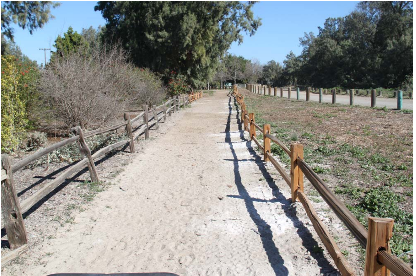
Lime from the old Cal Water treatment plant can be seen seeping up around the new fence holes in the Bird and Butterfly Garden of the Tijuana River Valley Regional Park.
