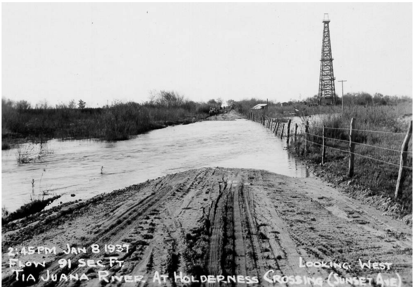
The derrick of the Holderness oil well is visible west of the Tijuana river on Sunset in 1937. (Photo courtesy of Sweetwater Authority)
