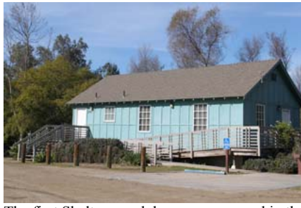
The first Shelton ranch house was moved in the 1990s, and is now the ranger building in the Bird & Butterfly Garden
