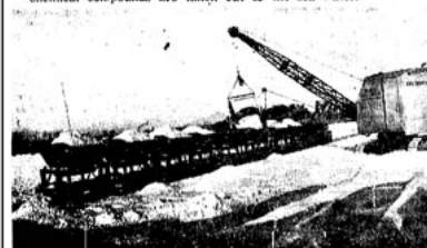
It looks like midwinter in Minnesota the year 'round during the '30s. The precipitated salt is gathered by a dragline shovel and loaded in gondolas to be hauled to the refinery.
