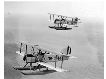
Douglas DT-2s from VT-2 at North Island
