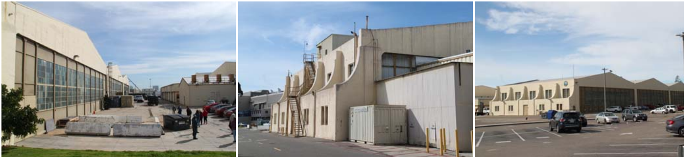
During 1918, Bertram Grosvenor Goodhue designed the first buildings in what is now the Naval Air Station Historic District, including these Seaplane Hangars (Buildings 1 and 2). More pictures of the district are at the NAS Tour page .
