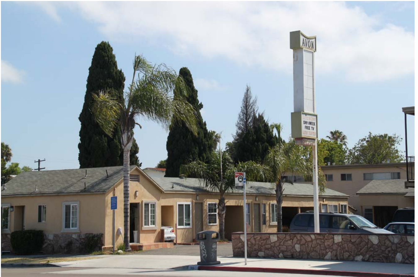
The Avon Motel at 99 Broadway in Chula Vista was originally the Chick Inn.
