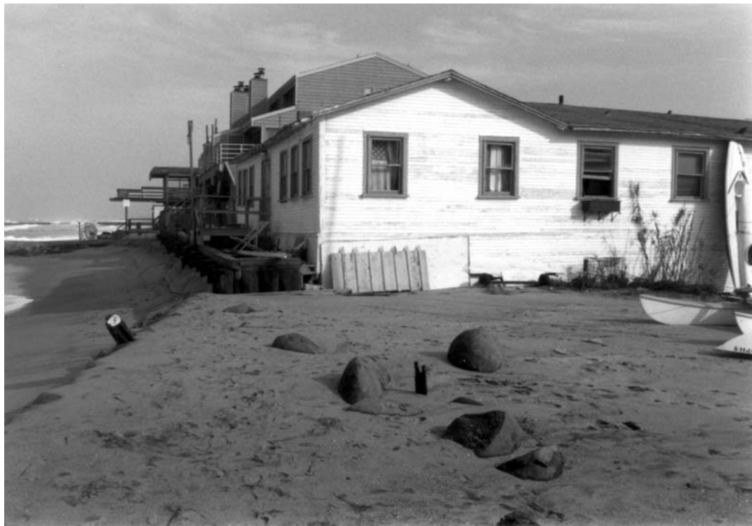
This photo looking north shows the "White House" in 1990 shortly before it was demolished. This house was built as a Children's Home in 1936 by Imperial Beach resident James O. Smith. During World War II it was a USO Canteen for servicemen. After the war Dempsey Holder lived in the house. According to the book Lifeguards of San Diego County , "The building was used as a crash pad for itinerant seasonal lifeguards and for the stray dogs that roamed the beaches of south county for years." One visiting Australian lifeguard exclaimed, "It's a flippin' surf hole!" (Photo courtesy of City of Imperial Beach Lifeguard Service.)
