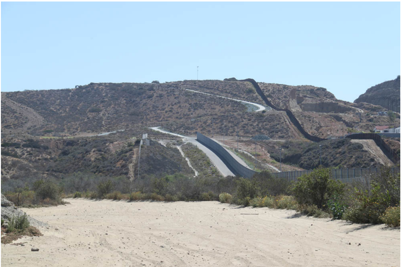
The triple border fence ends at the base of Bunker Hill, looking east from the base of Lichty Mesa in 2015.
