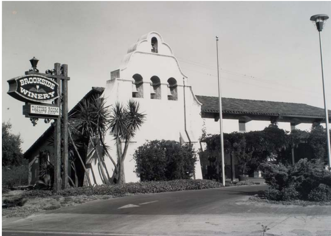
Designed by local architect Victor Wulff and inspired by the California Missions, the Brookside Winery Tasting Room was finished in 1965. It was at a meeting at the Tasting Room that the Bonita Business and Professional Association (BBPA) was born. The Tasting Room operated until the 1970s when it was remodeled for the North Island Credit Union. It is now the Performance Cyclery. (Photo from the Bonita Business and Professional Association.)
