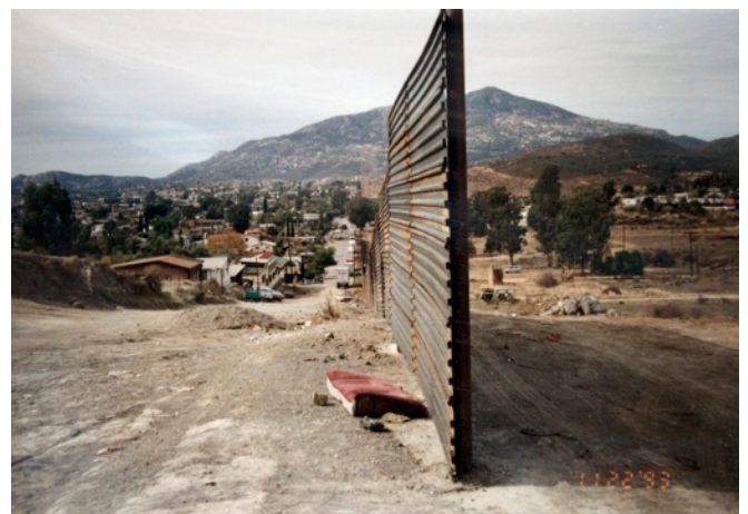
Surplus military landing mat being installed in 1993.
